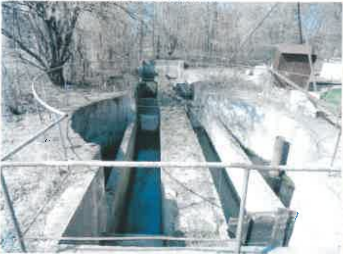
Statie epurare decantare clorinator
