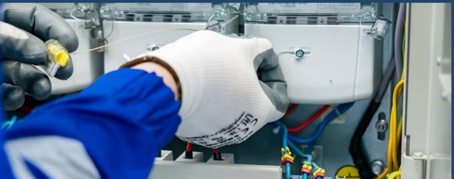
Premier Energy smart meter installation in the Republic of Moldova.
