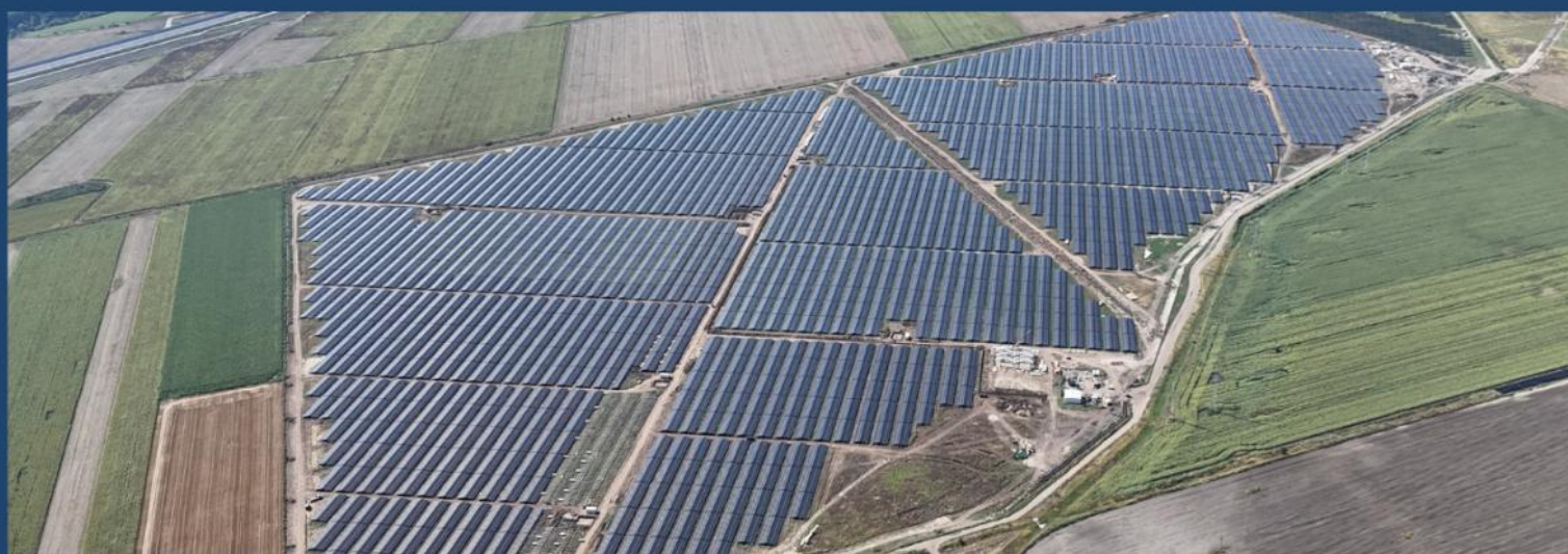
Premier Energy's 48 MW solar park development with a battery storage capacity of 16 MWh in Stalpu, Buzau County, Romania.
