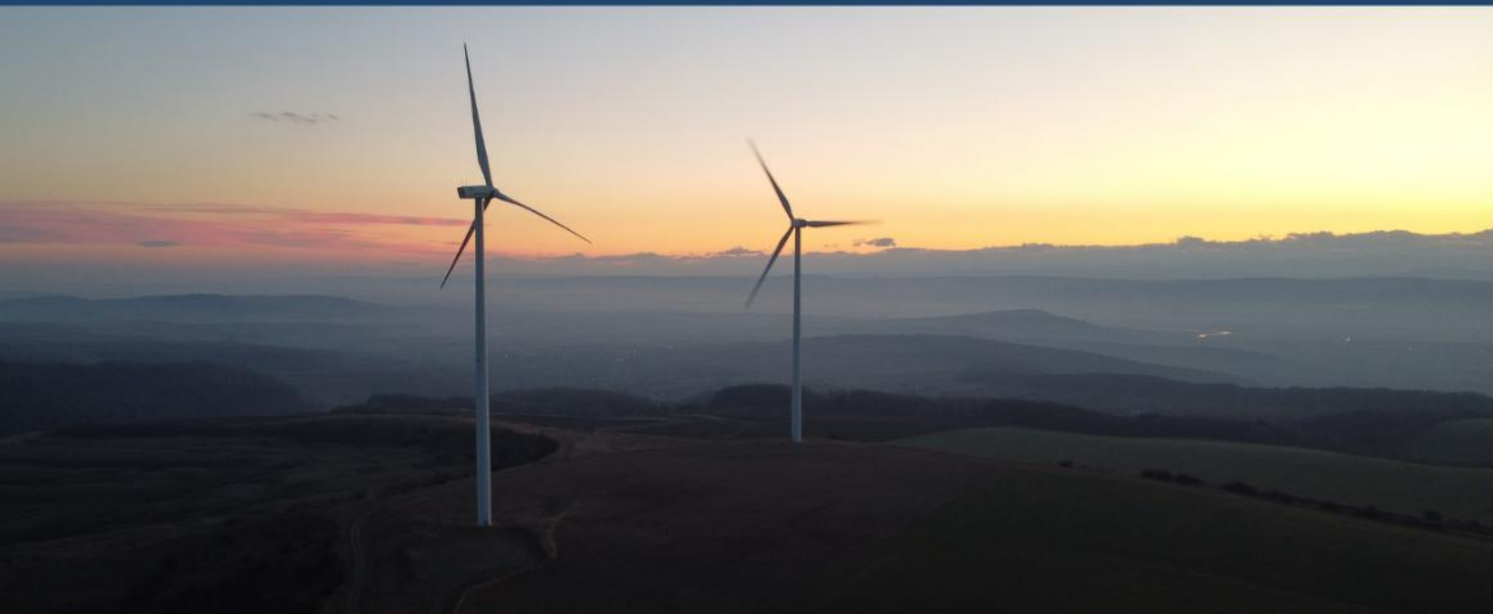
Premier Energy's 18 MW wind park near Drancenii, Vaslui County, Romania.
